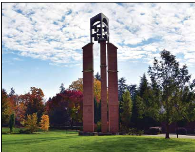
The University of Oregon plans to remodel the interiors of buildings purchased from Concordia University. Some students may arrive on the Northeast Portland campus later this year. (University of Oregon)
