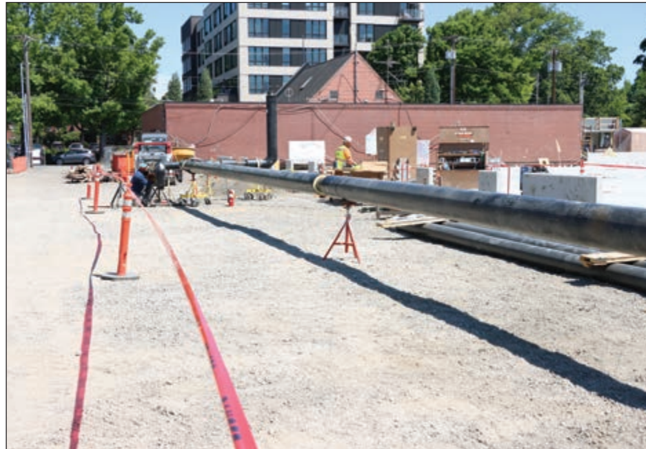
The plumbing system at Benson is being replaced, along with its electric system. (Portland Public Schools)
