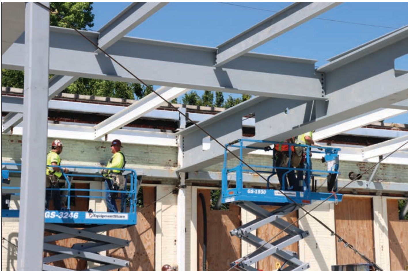
Construction crews work on upgrades at Benson Polytechnic High school. Renovations include seismic retrofitting and new, two-story wings for Career Technical Education and core academic learning spaces. (Portland Public Schools)
