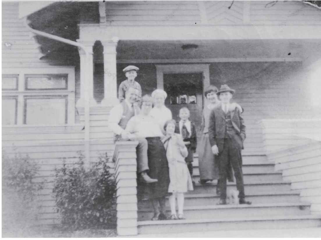
The Morrison family gathered on the porch of their Alameda home in the early 1900s. Doug Decker, who started the Alameda Old House History blog, now lives in the house. With the help of the historic photo, he rebuilt the porch to mimic its original look.
