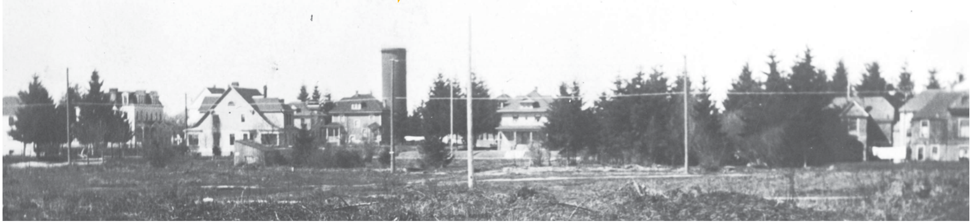
A pre-1906 photograph shows the water tower standing at Northeast Schuyler Street and 13th Avenue. It held 350,000 gallons of water. (Photos courtesy Oregon Historical Society)
